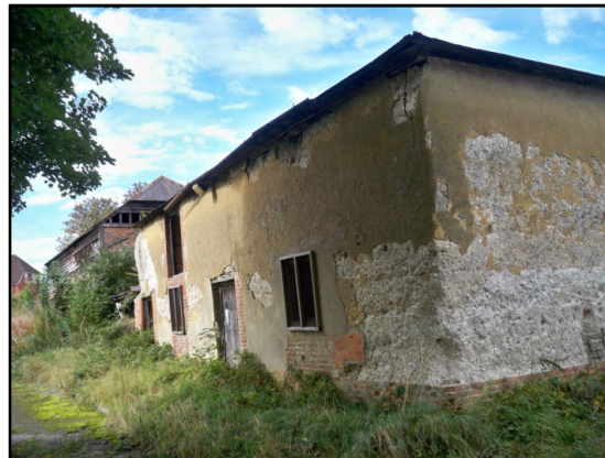
Cob barn to be demolished
